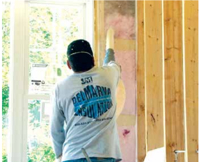
R-23 BLOWN-IN INSULATION
